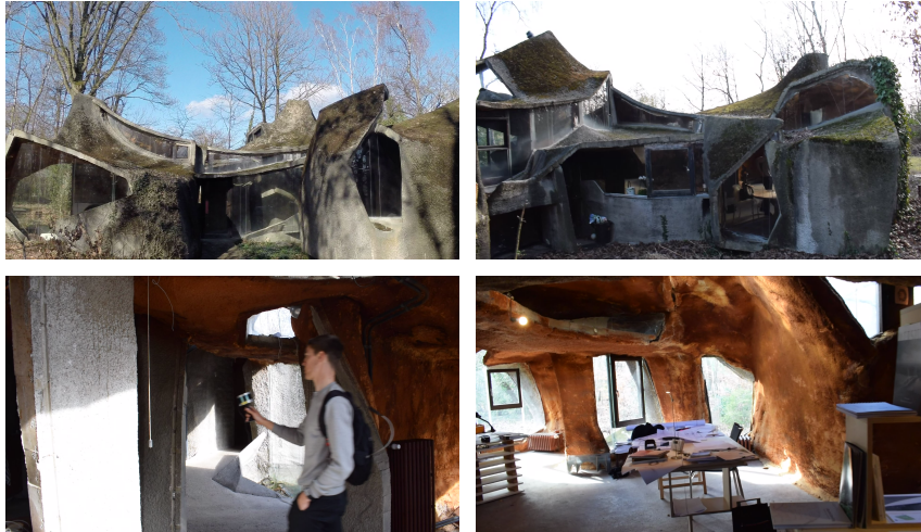
Figure 7.15: The extraordinary shaped sculpture house Gillet in Angleur. The house was built using shotcrete, a.k.a. sprayed concrete, which allows the walls to be irregularly shaped. The lidar scanner was hand-held during acquisition because the floor had too many irregularities for Liborg to be able to move around.
