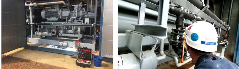
Figure 8.2: The cooling container that was the subject of an AR-applications supporting its maintenance. Maintenance instructions can be virtually attached to an object of interest in the real world.
